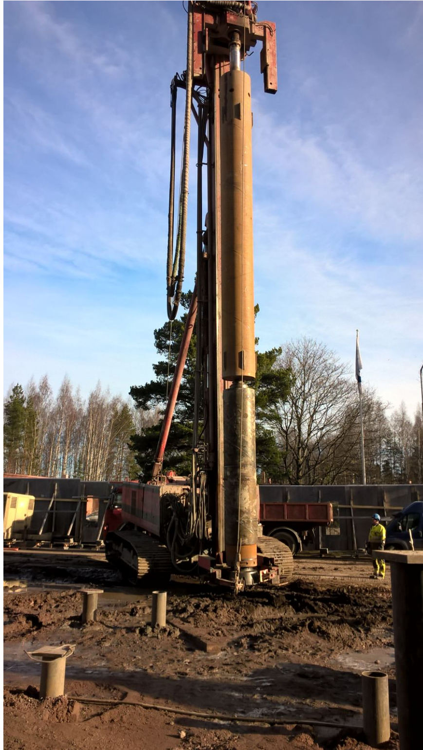
Picture 7.3: Example of 30" diameter air hammer bit equipped with large diameter drill collar to make the area smaller. The 42 m deep conductor sections were made with this equipment in Otaniemi project.
